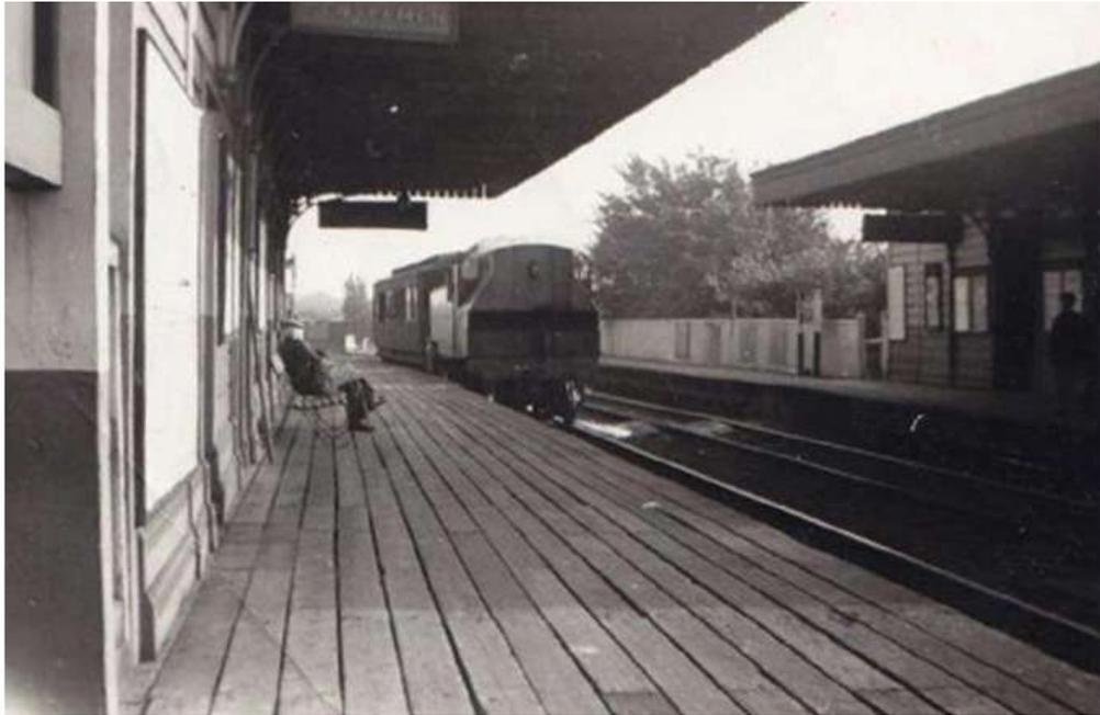
*Parkgate station with what appears to be an Ivatt-designed LMS class 2 2-6-2 tank engine, waiting for the signal to clear, operating a push-pull service to Hooton with an old clerestory coach. The seated gentleman, posed for the photo, seems to be here to watch the trains rather than take one. The signs hanging from the canopies indicate the position of the pedestrian subway, while the gap in the fence marks the start of the path leading down to the Ropewalk.*
