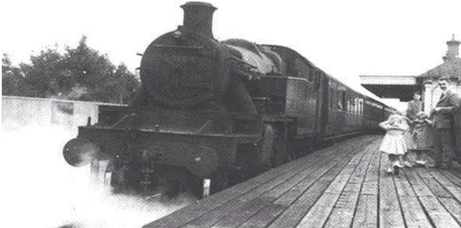
*At Parkgate Stanier-designed LMS class 3 2-6-2 tank engine No 40144 heads a train for Hooton; the small children block their ears against the noise of escaping steam.*
